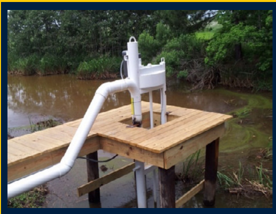
OUR 6" PUMP CAN TOLERATE 2" SOLIDS
